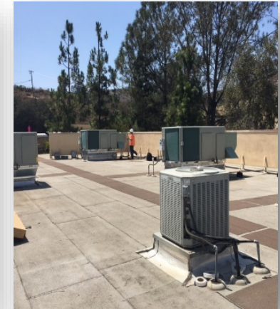
Cuyamaca College Building L HVAC Unit Delivery
