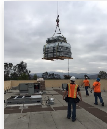
Cuyamaca College New HVAC Units on Building L
